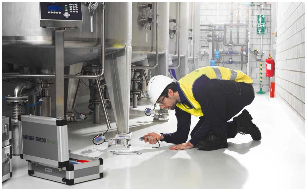
Access to load cell for cleaning, inspection and maintenance is convenient because they are at the bottom of the tank and never in contact with material stored inside tank.
