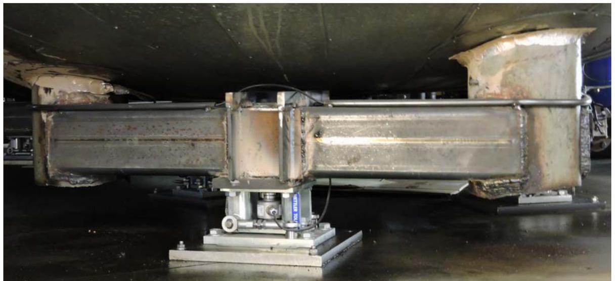
On this tank a bio lubricant manufacturer modified the tank's legs to integrate weigh modules for replacing flowmeters. This change made it easier for him to achieve high quality goals during filling and formulation. In addition, more reliable and accurate inventory control allows for better management of expensive raw materials.
