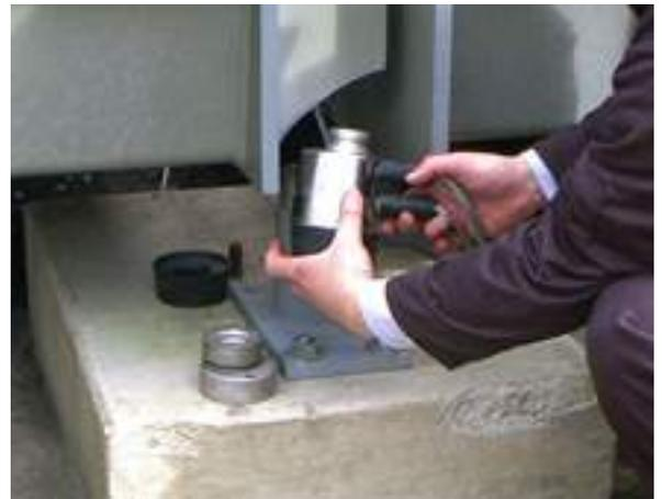
Periodically check load cells, receivers and other critical parts for wear
